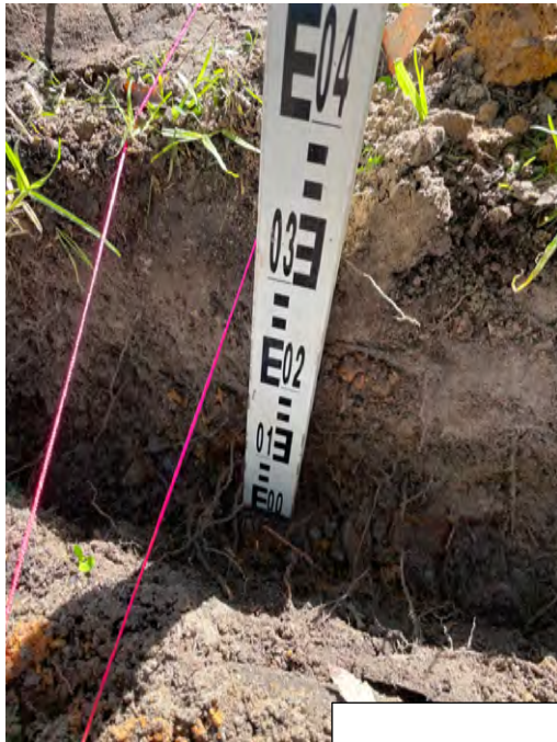
Images showing trench and trench depth.
