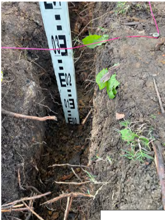
Images showing trench and trench depth.
